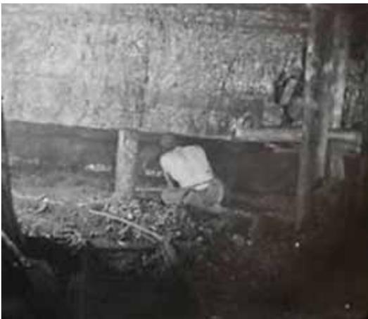
As the hewing nears completion the coal that is on the brink of collapse is termed as being “ripe”.
