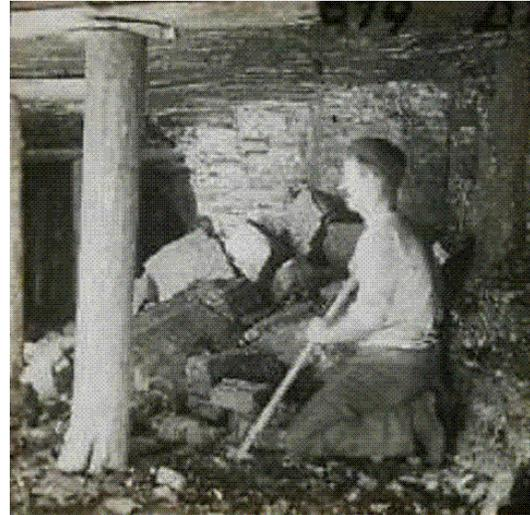
Removal of the temporary sprags allows the undercut face to collapse, breaking up the rock along the coal’s cleat into manageable blocks of coal. The next issue of this Newsletter will show some slides relating to underground transport and haulage.
