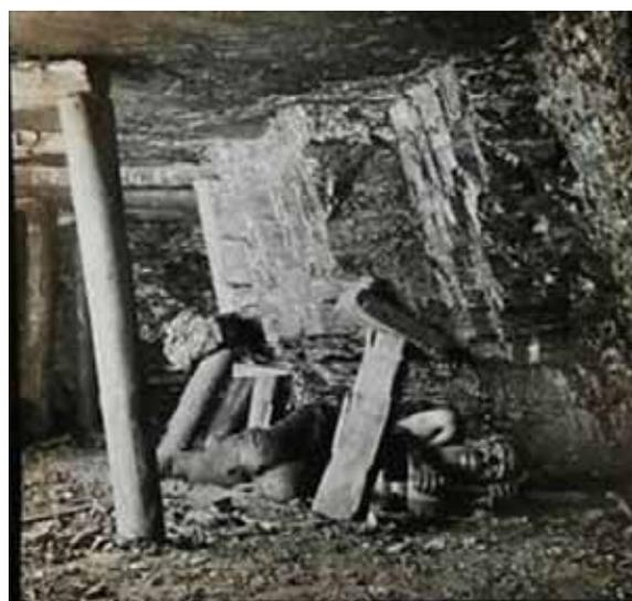
To the left of the picture is a standard pit prop, offering support to the roof of the “stall”, spanning between floor and roof. The shorter temporary timber supports that the collier is working behind are called “sprags”.
